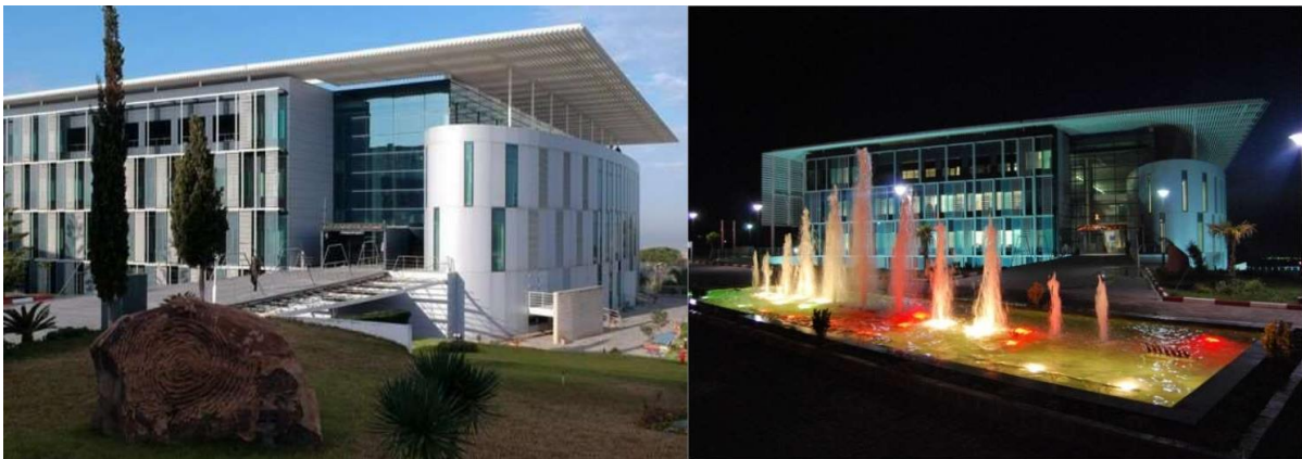
NICC/NG main building
